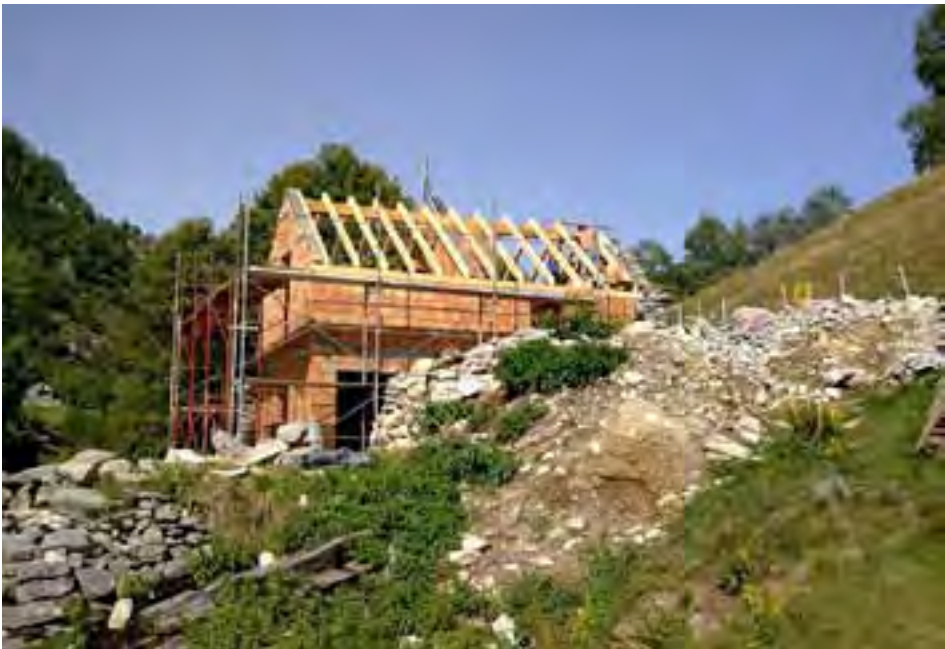
• The new rustico under construction, with the chestnut ridge beam.
